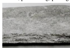
Figure 1 Asbestos-containing construction material
