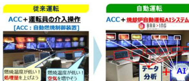
Fig.1 Image of incinerator operation of WtE plant
