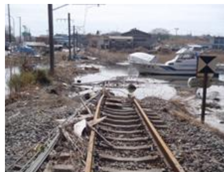
Fig.3 Washed away of track
