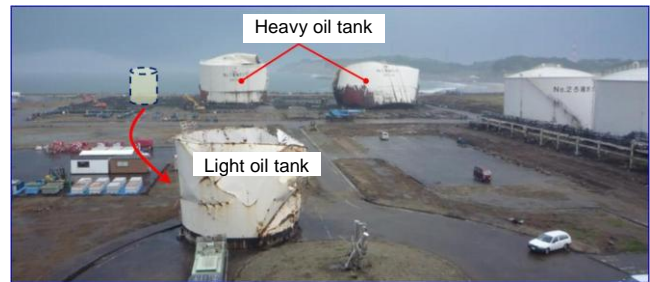
(b) Damaged light and heavy oil tanks.
