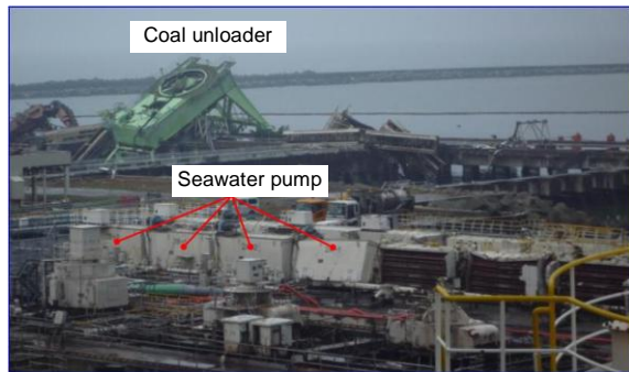
(a) Damaged coal unloader and sea water pump.
