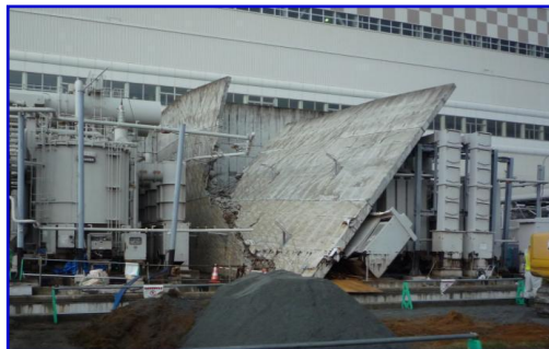
(c) Damaged concrete wall.
