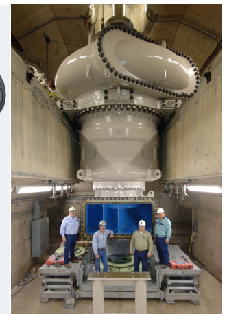
Fig.2 Completion of the pump assembly
