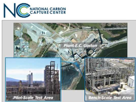
Figure 1. Photographs of Post-Combustion Carbon Capture Test Facilities
